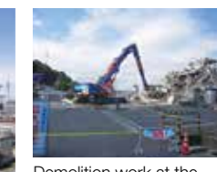
Demolition work at the Matsuyama Plant
