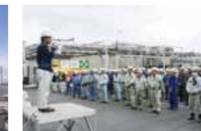
Safety rally on the first day of periodic repair work
