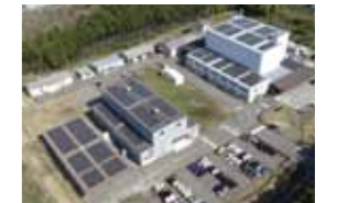
Installing photovoltaic panels on rooftops
