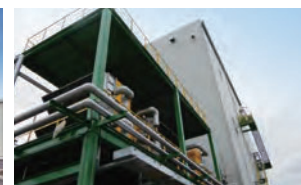
Constructed an optical polymer manufacturing plant
