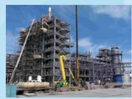
The Netherlands (MXDA/Under construction)
