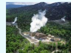
Geothermal power generation
