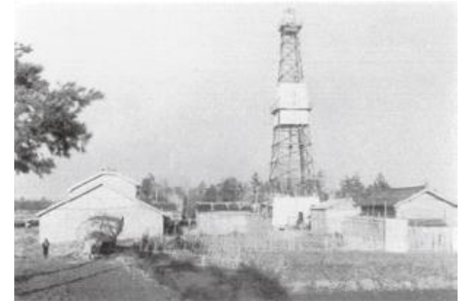
Water-dissolved natural gas well excavation during initial development
