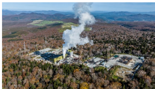
Appi Geothermal Power Plant Source: Appi Geothermal Energy Corporation
